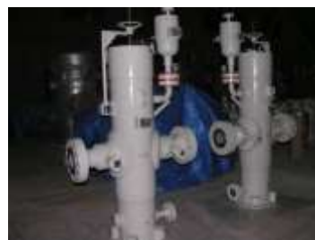
Fabricated Basket Strainers with Air Eliminators (FAB-SAE)
