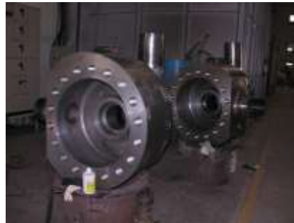
Welding work on Nuclear Shutdown cooling Pumps
