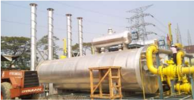
INDIRECT FIRED WATER BATH HEATERS FP-IFWBH
